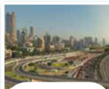
MUMBAI COASTAL ROAD MEGA PROJECT
