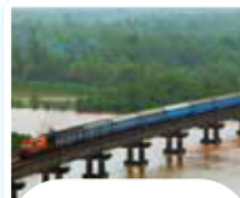
KONKAN RAILWAY PROJECT
